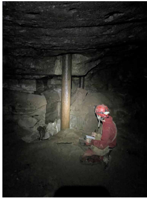
Figure 3. Drainage well casings in the Breakdown Canyon section of Hidden River Cave.
