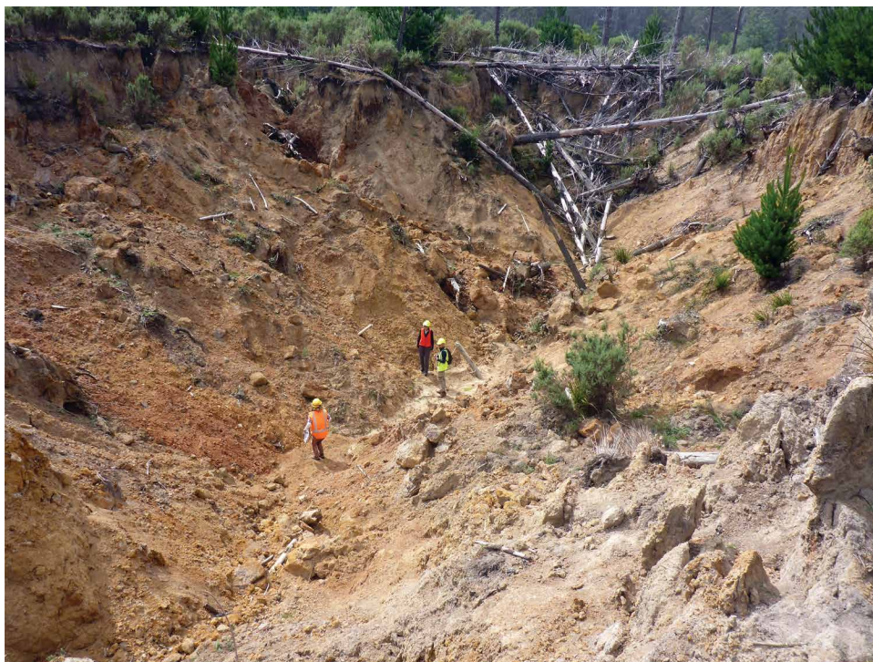
Figure 3. Sinkhole 1 in March 2019. This sinkhole formed in the winter of 2016 when several smaller sinkholes formed in 2013–2015 coalesced. It is the largest in the study area at over 60 m wide and 10 m deep with a footprint of 1450 \text{m}^2 . An estimated 6000 \text{m}^3 of soil derived from Quaternary deposits have been lost to the underlying karst at this site. The furthest figure is standing on an exposure of limestone bedrock with a small cave entrance into which runoff flows during heavy rainfall.
