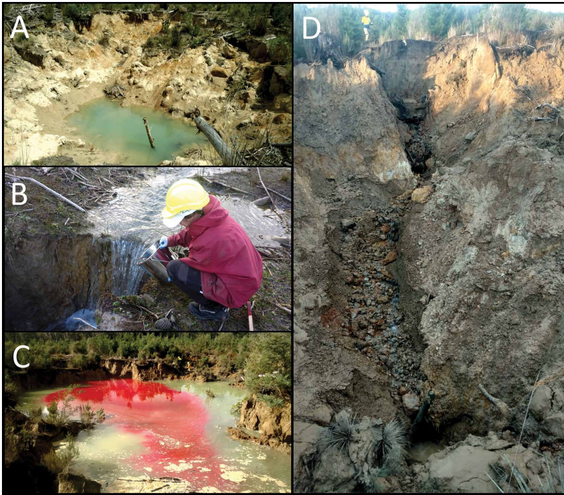
Figure 7. A. After heavy rain a lake (informally named Blue Lake) forms in Sinkhole 4 (photographed October 26, 2017); a small stream. B. (estimated flow 5–7 L/s) originating from a flooded Eastern Creek flows into it (photographed 26 July 2018). C. 870 g of Rhodamine WT dye was injected into this stream on July 26, 2018. D. By the afternoon of Saturday July 28, 2018 the lake had completely drained and the stream was seen cascading into an unstable vertical shaft at the base of the sinkhole which was over 7 m deep. The shadow line marks the approximate previous water level as shown in C.
