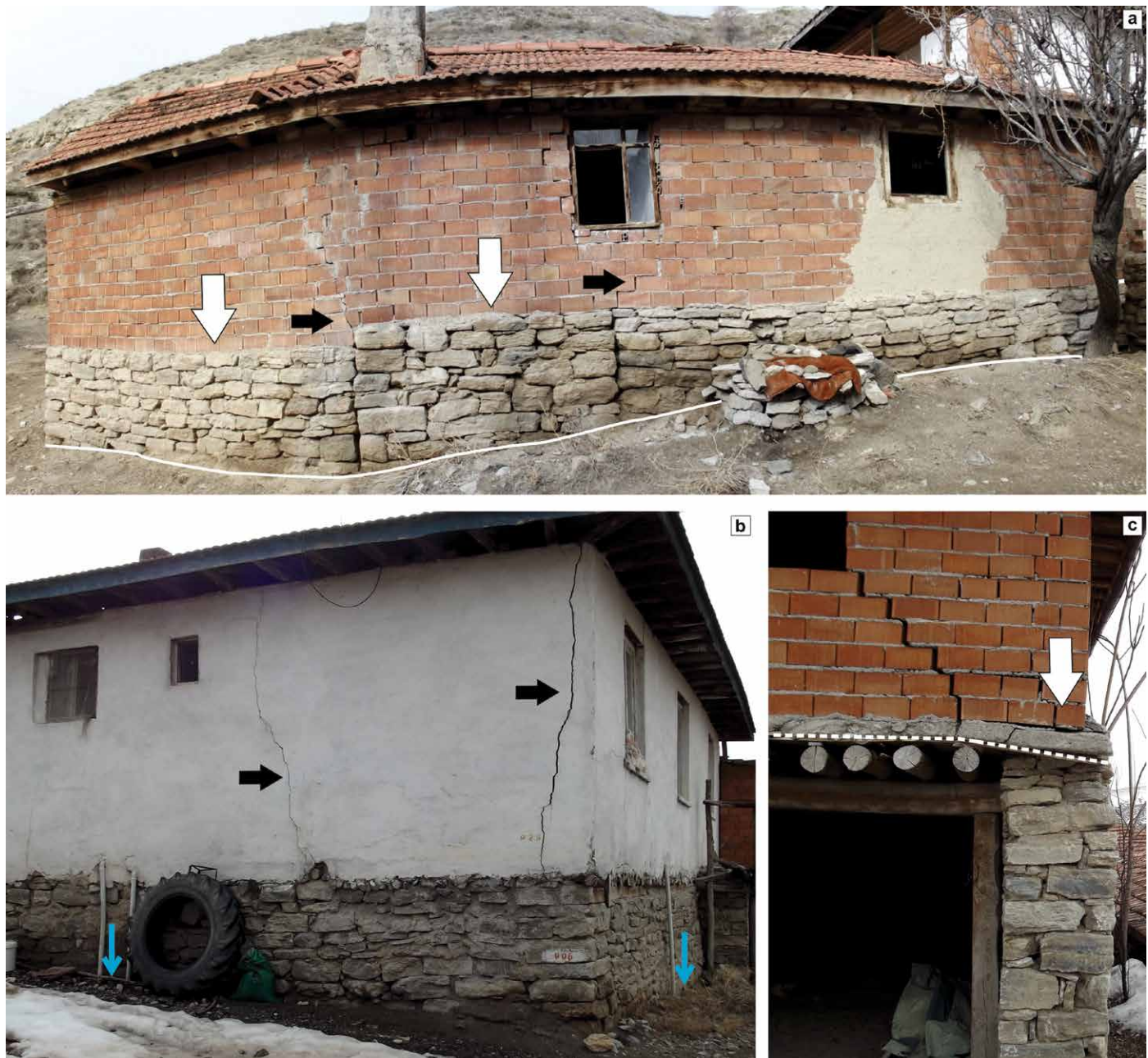
Figure 4. (a) Displacement of house wall showing bulging and cracking caused by subsidence, and broken windows due to distortion. (b) Cracks on wall and pipes draining wastewater directly into ground. (c) Open joint in wall of building. (Photographs taken on February 26, 2017).
