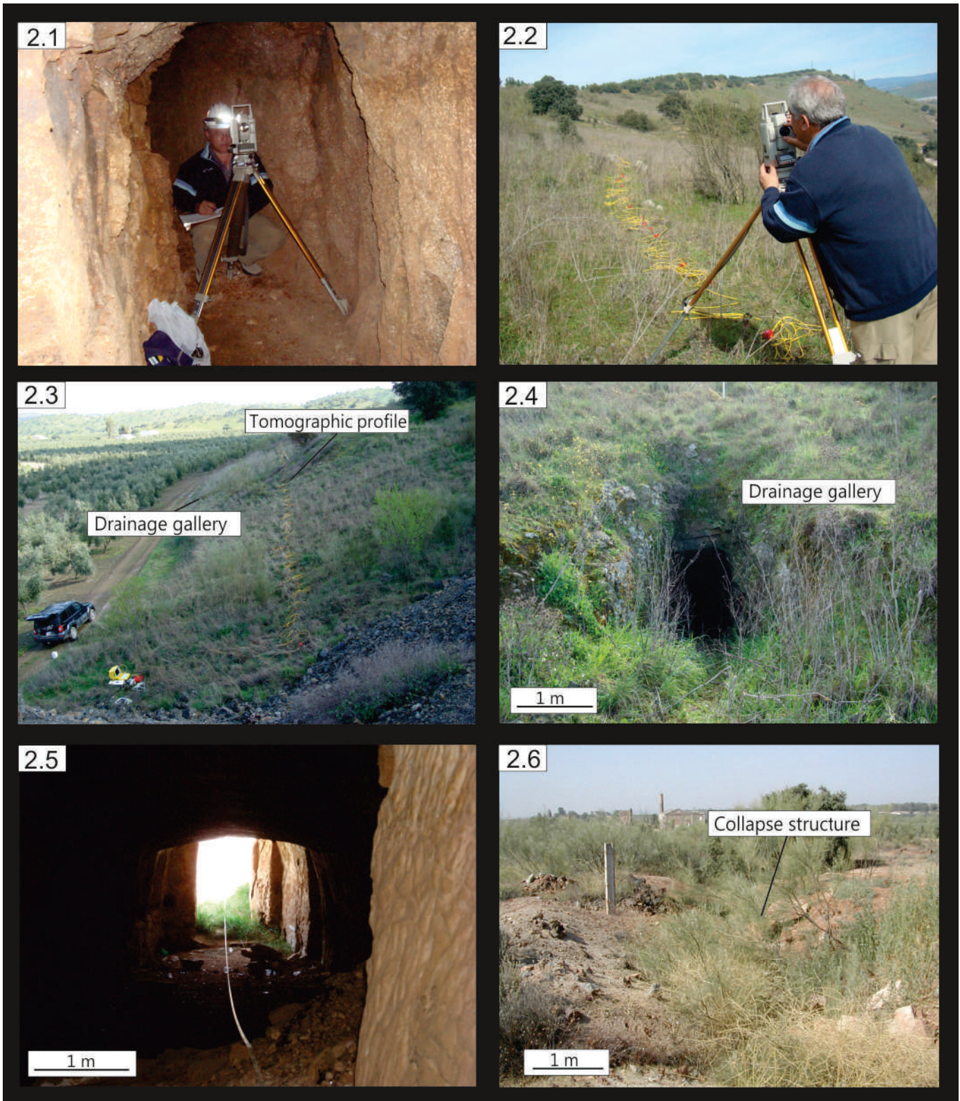
Figure 2. 2.1: Surveying inside the drainage adit at site A, the Mimbres Cavity. 2.2: Topographic surveying at the surface above the tomography profile at site A. 2.3: Route of the electrode array at site B, the Grupo Cobo Cavity, and the entrance to the drainage gallery. 2.4: The entrance to the drainage adit at site B. 2.5: Interior of the mine tunnel that is site C, the Canena Cavity. 2.6: Collapse associated with the caved seam at site D, the Arrayanes caved seam.
