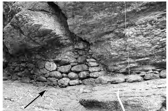
Figure 6. Old dry walls, built to waterproof the Rio Garrafo stream bed.
