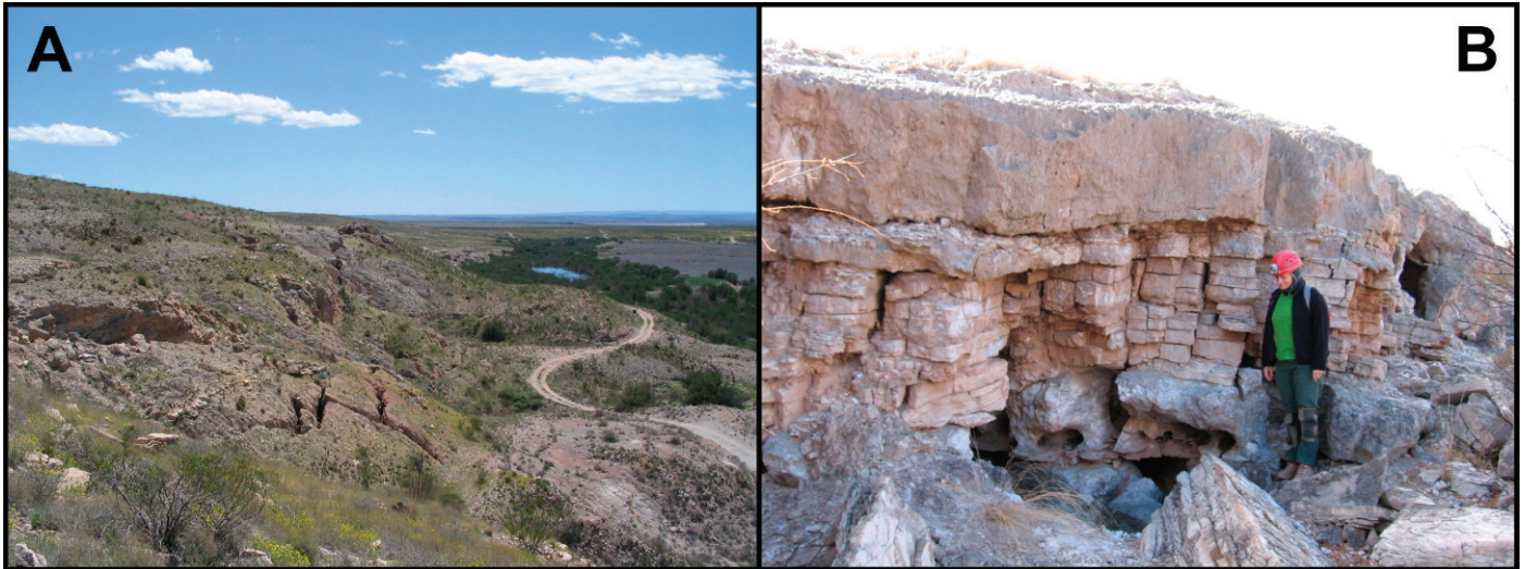
Figure 7. McMillan escarpment showing large earth fissures (A) and complex entrance network (B).
