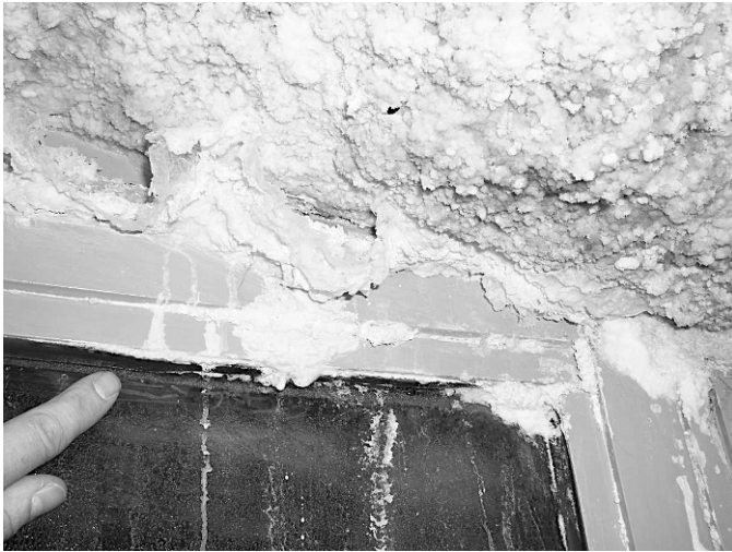
Figure 5. Detail of the frame of the glass door. Aluminum sulfate crystals are growing on outer side on aluminum frame, along rubber joints. Outside temperature is 24 °C, inside temperature is 37 °C; humidity at saturation produces condensation on the glass.
