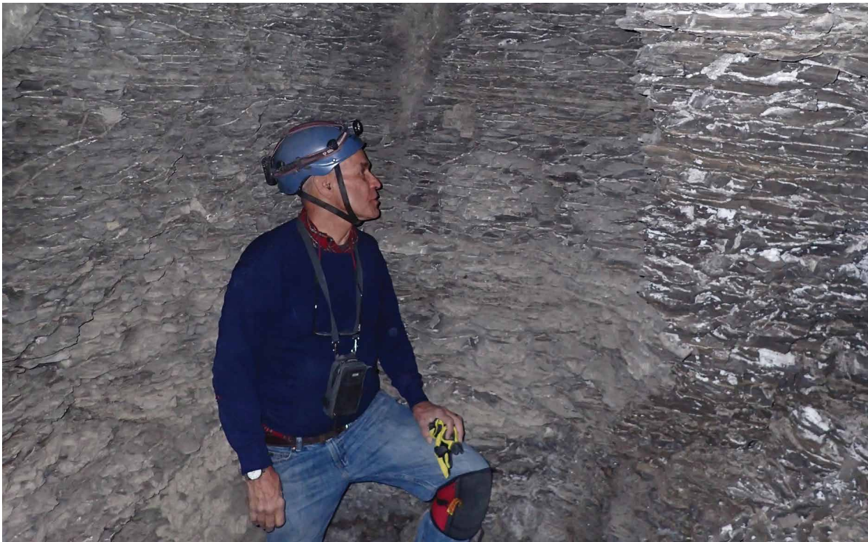
Figure 13. Gypsum fracture fillings in passage wall.
