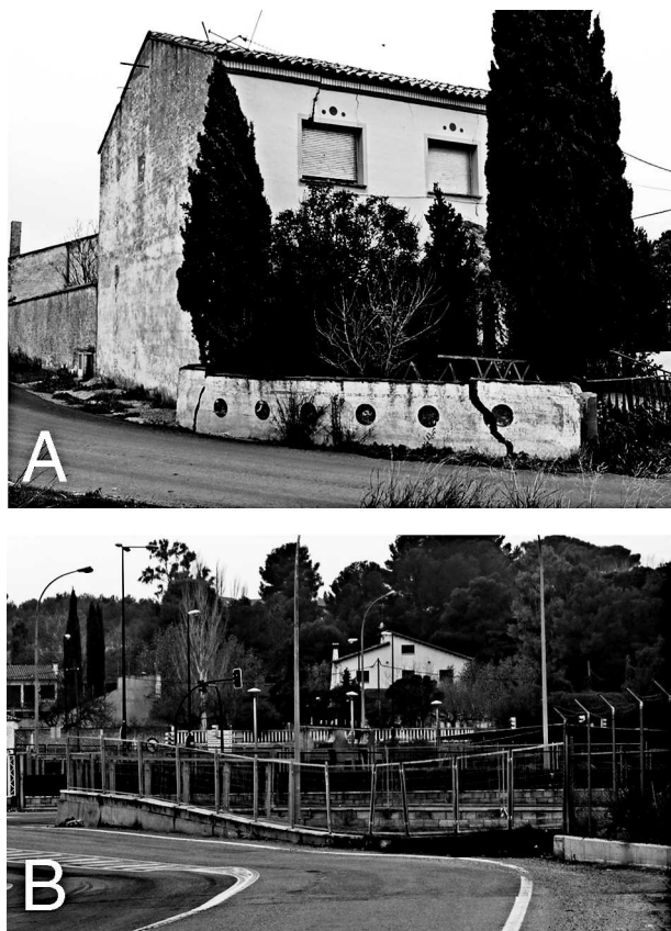
Figure 4. Damage in urban areas northwest of the city of Zaragoza resulting from karst subsidence. A, fractures in walls. B, strong deformation of a fence.
