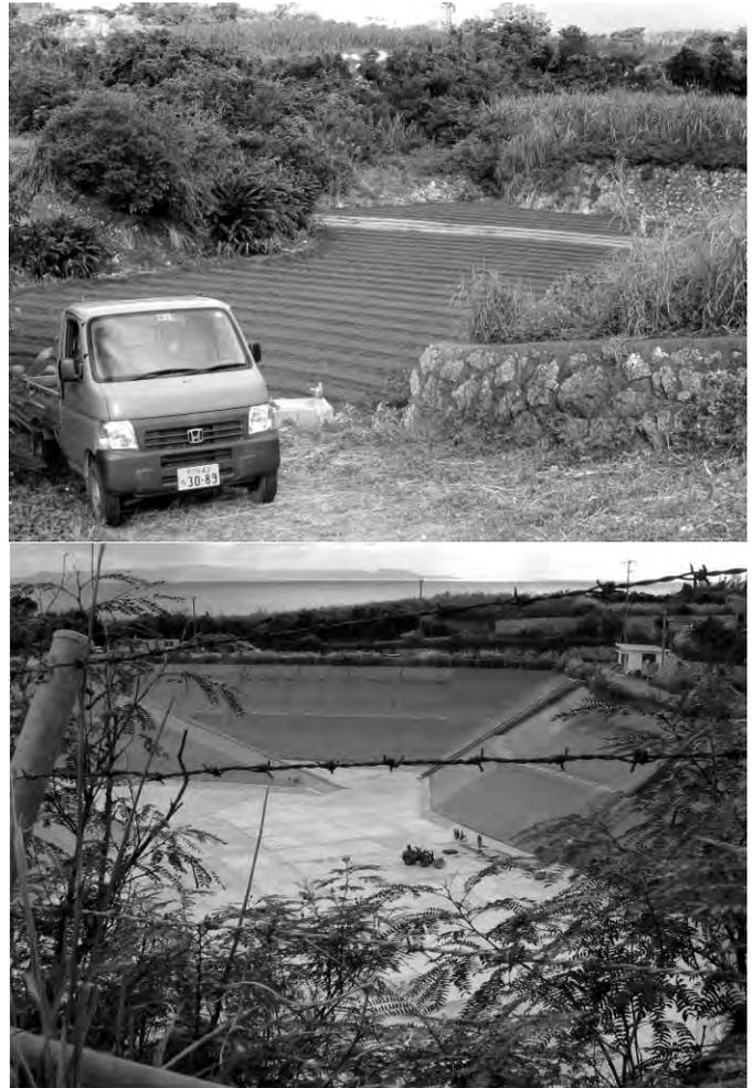
**Figure 3. Top: Typical small shallow depression on Yoron; most closed depressions are used for agriculture. Bottom: Excavated and lined depression to be used as a water reservoir for irrigation.**
