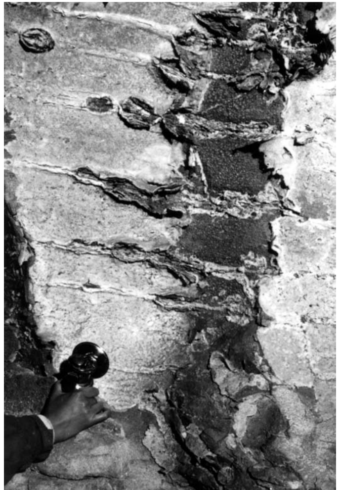
Figure 2. Wall of Turner Avenue showing extrusion of gypsum along bedding planes.
