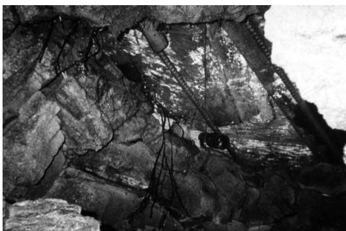
Figure 3. Looking diagonally upward to a pipe connected directly to a toilet in north Puna District, near Keaau. A pile of moist feces was present beneath the pipe.
