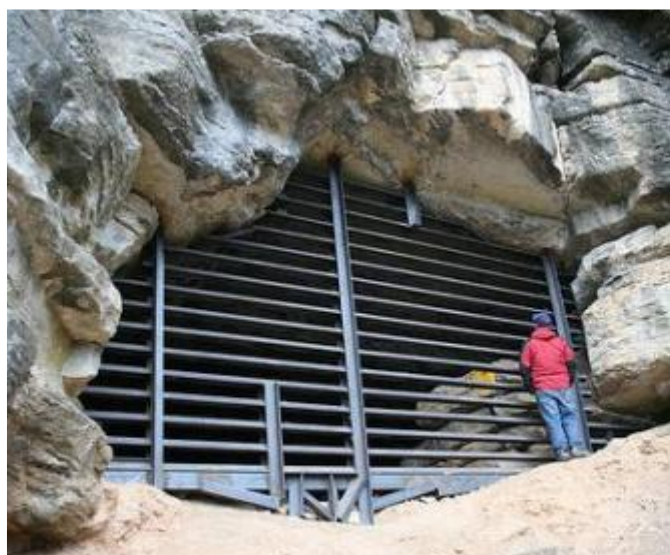
Trout Cave after it was gated in Fall 2008 to protect Indiana bats. Photo by Brian Masney
