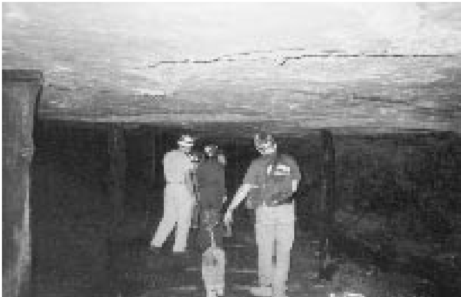
Exploring through the Utica Cement Mine. Photo by Troy Simpson
