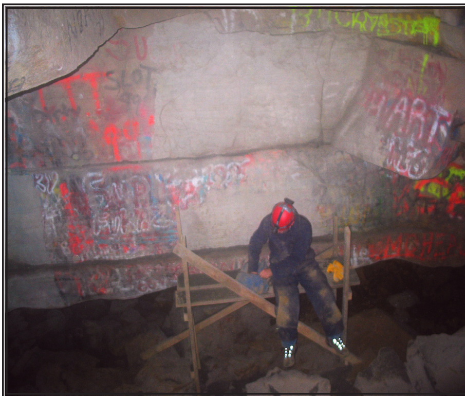
The effectiveness of sandblasting can clearly be seen in this photo by Ralph Sawyer.
