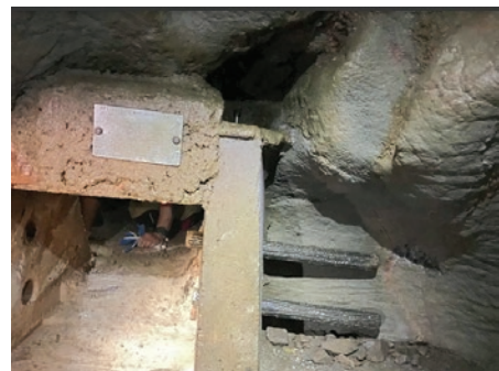
The new inner gate at Bells from the inside showing locking bars in open position and instruction plaque for upper bar release
